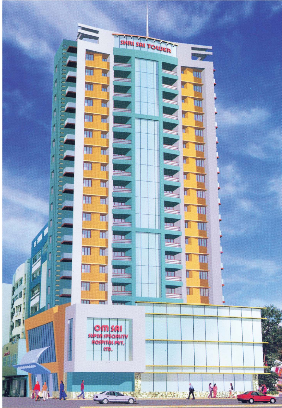
“Shree Sai Tower” Nutan Nagar, Sodawala Lane, Borivali (W), Mumbai.
