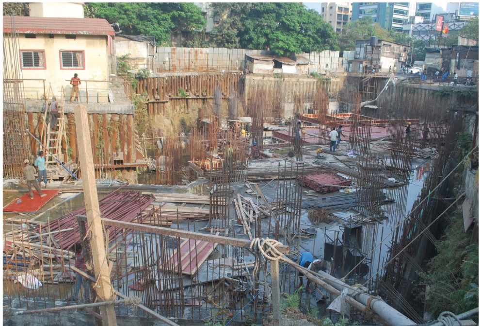
“ Tulsi Chamber” (Work in progress) Opp. Swastik Chambers, Chembur, Mumbai
